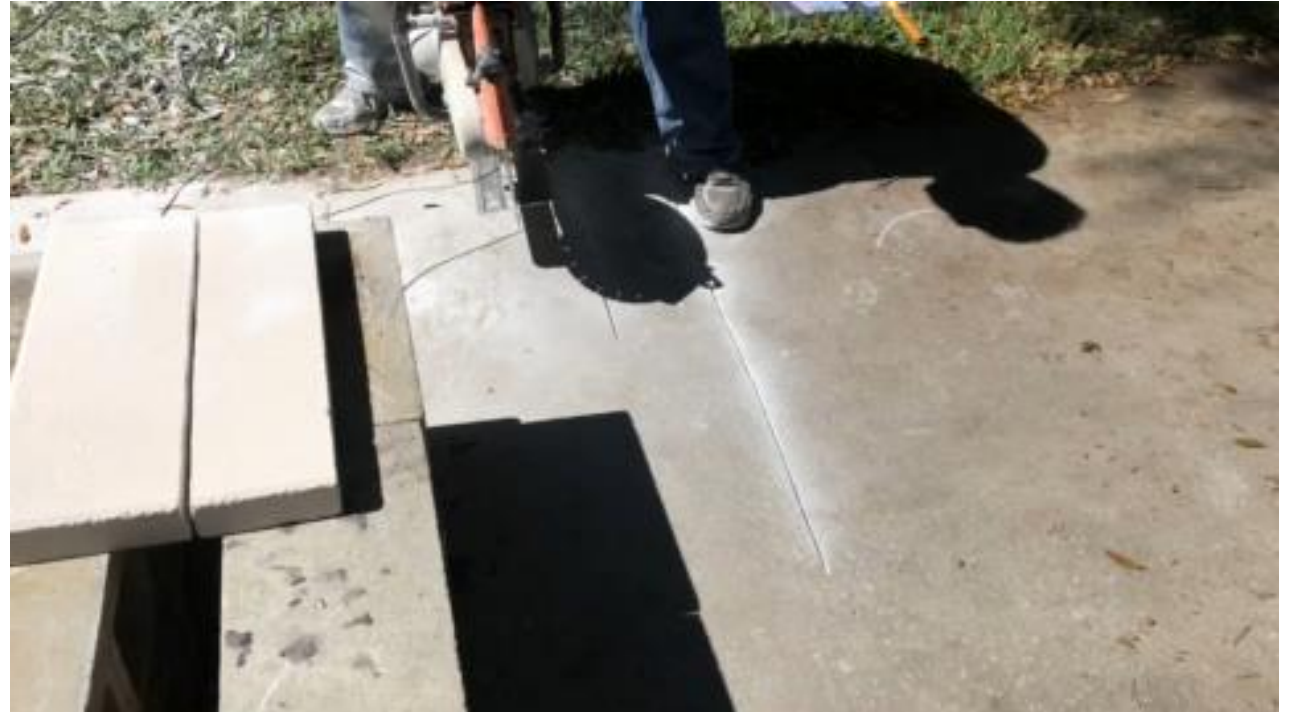
Figure 1. Video of the test procedure for the Lones Stone Saw. Cuts were made into a poured concrete driveway both with and without the Lones Saw Shoe.
